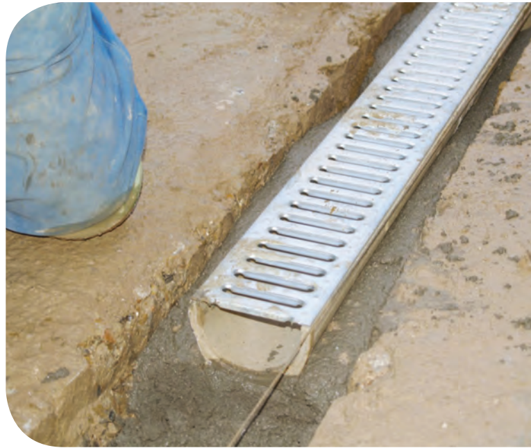
Installation of drainage channels, webercem pyracrete
