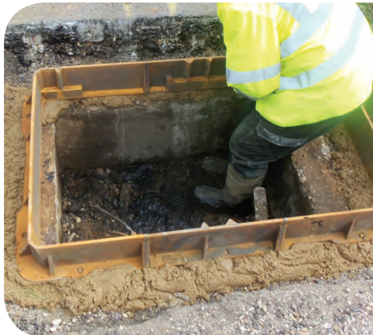
webertec bedding mortar haunching
