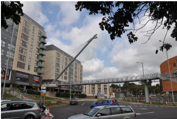
Hemel Hempstead Footbridge
