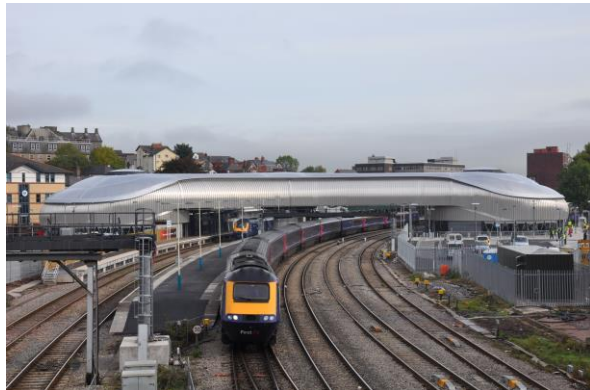
Newport Station Hub and Footbridges
