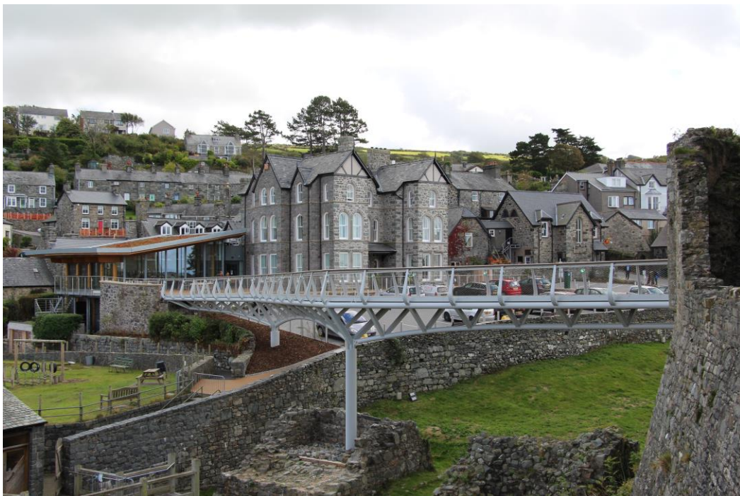
Harlech Castle footbridge
