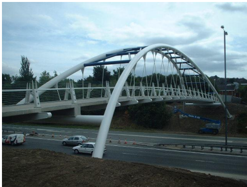
A57 Parkway Footbridge Sheffield
