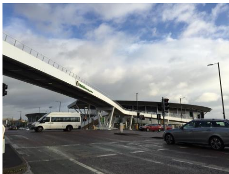
Manchester City FC Link Bridge
