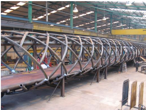
90m span bridge being assembled
