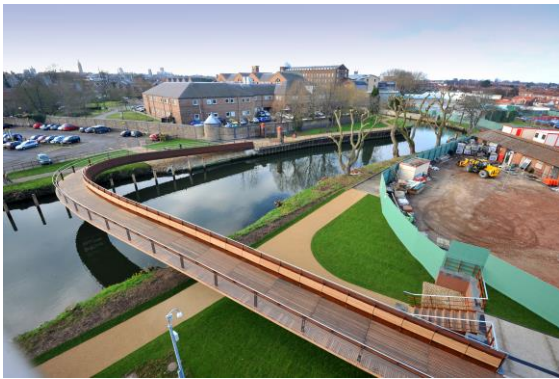
Jarrod's Footbridge, Norwich
