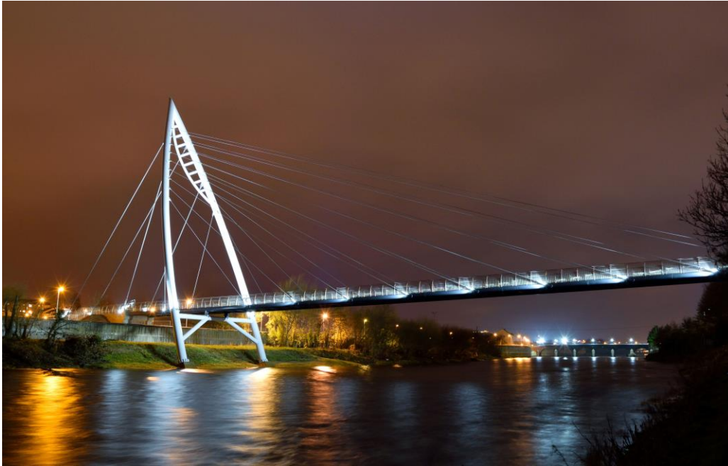
Strabane Cable Stay Footbridge N.Ireland
