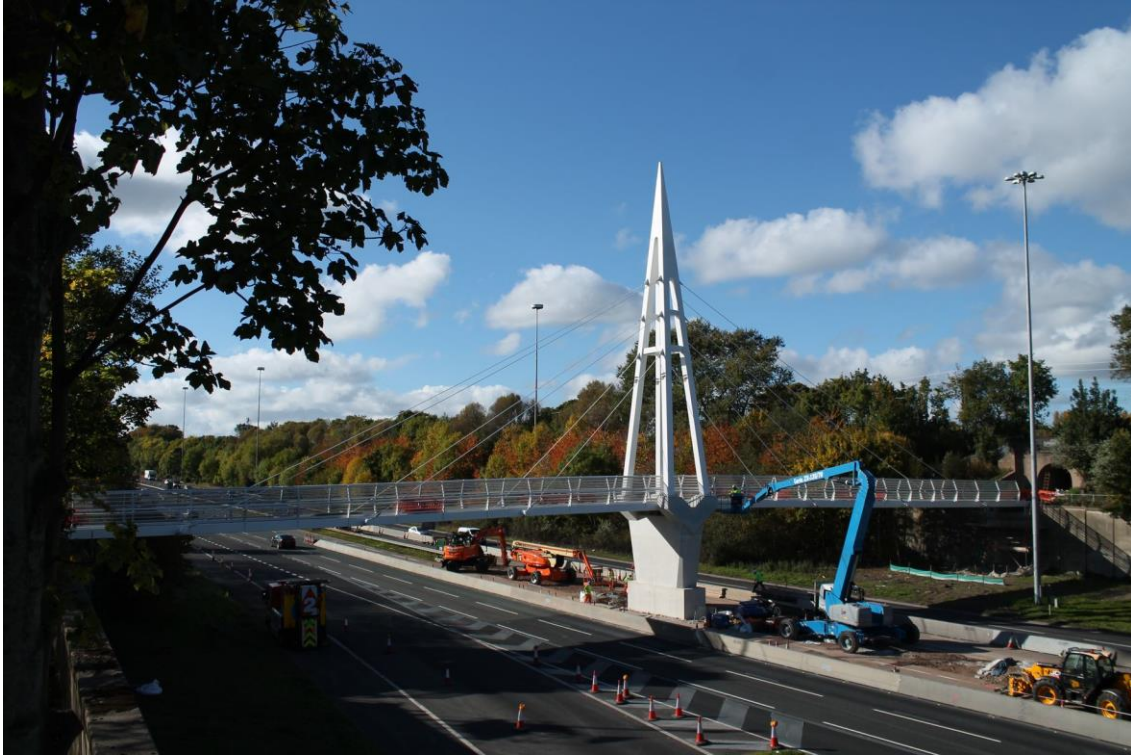
M62 Greystones Bridge
