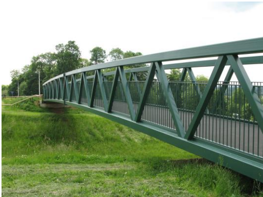
Sustrans Footbridge, Scunthorpe
