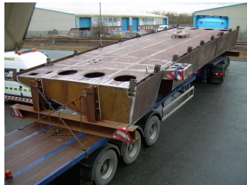
Completed plated bridge deck leaving works
