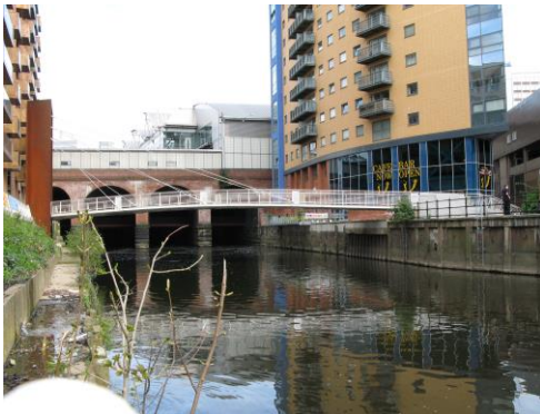
Waterman's Footbridge, Leeds
