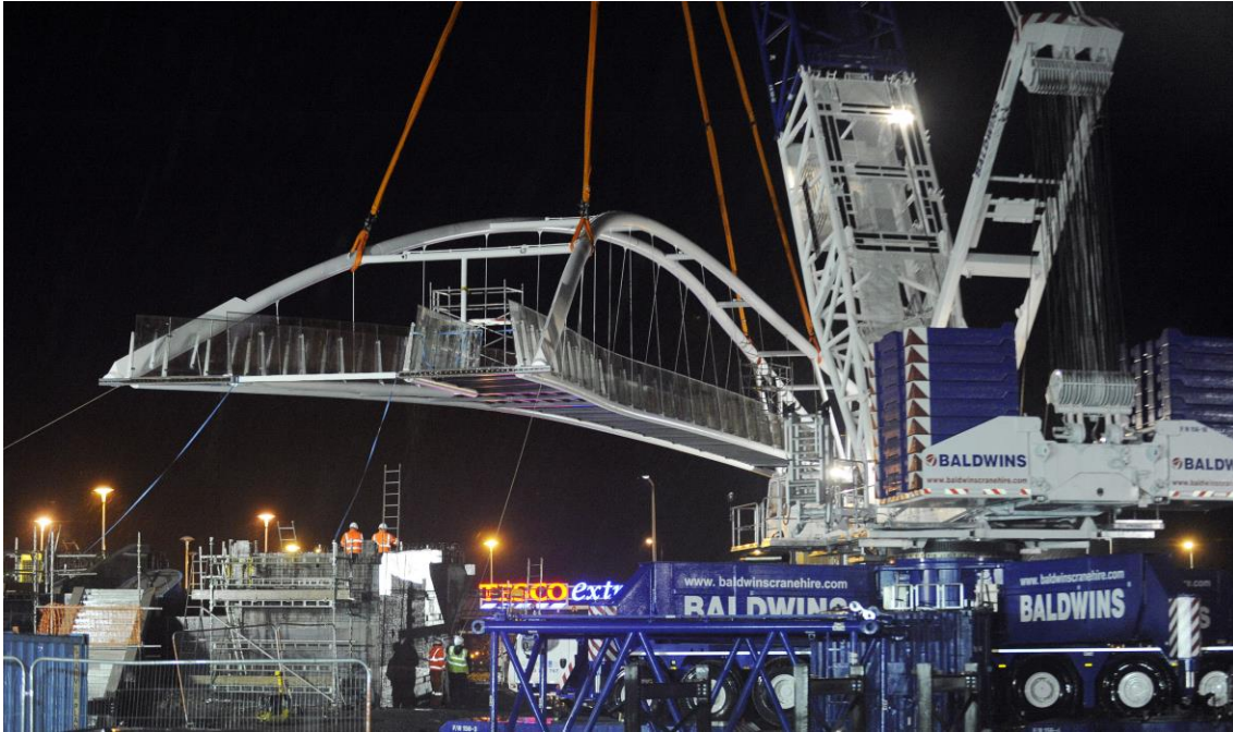
Seabraes Footbridge, Dundee
