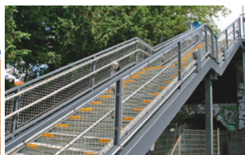
Metallic objects: balustrades, fences, railings, shelves, doors, etc.
