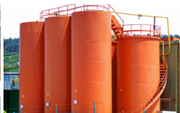
Reservoirs: silos, oil tanks, water tanks, etc.
