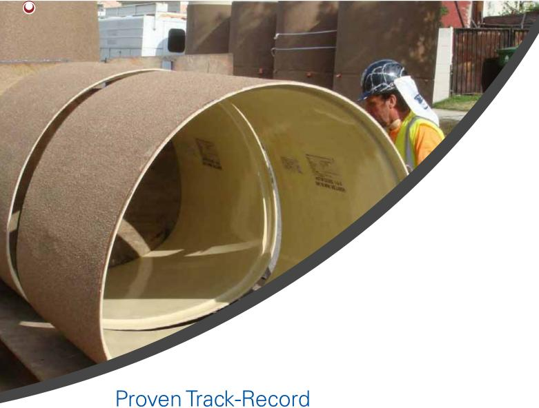
The Channeline GRP Structural Lining Systems have a proven track record for large diameter pipeline rehabilitation around the globe. Channeline products have been installed in projects in more than 30 countries worldwide.
