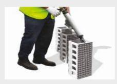
**3.** Envirodeck sealant is applied around the end of the unit prior to placement.
