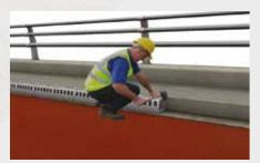
**4.** Place Envirodeck unit on the prepared mortar bed using a rubber hammer for adjustment to line and level.
