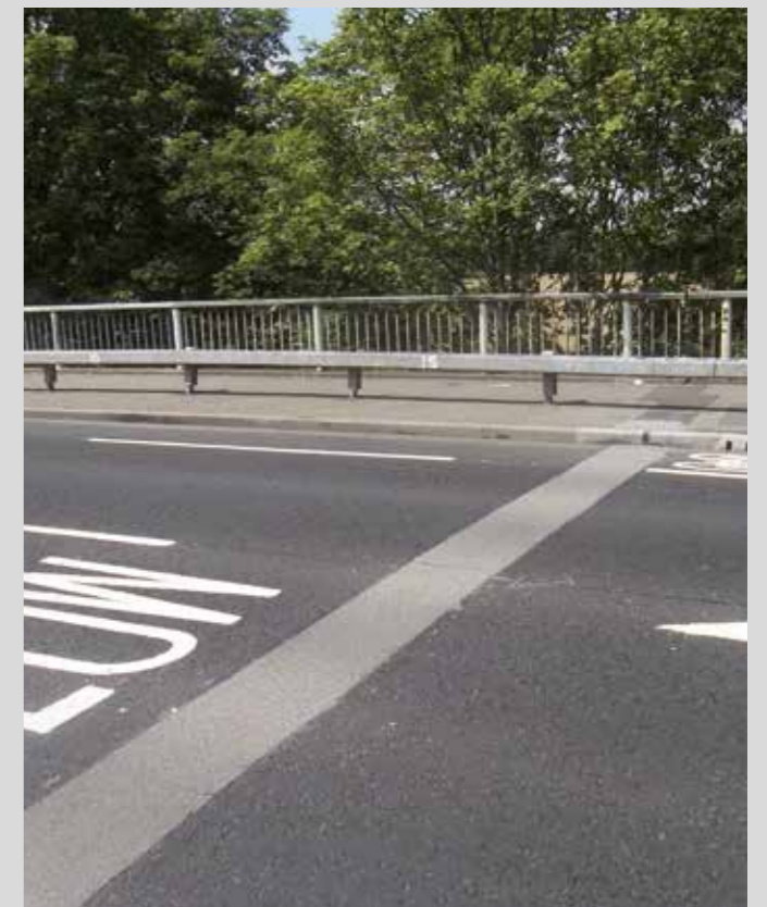
FEBA joint extends across the full length of the carriageway and into the verges.
