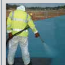
Bridge deck Waterproofing
