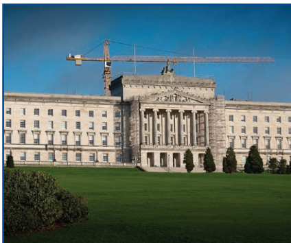
Stormont, Northern Ireland Roof slab protection
