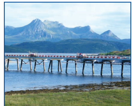
Kyle of Tongue Bridge, UK Pre-stressed beam protection
