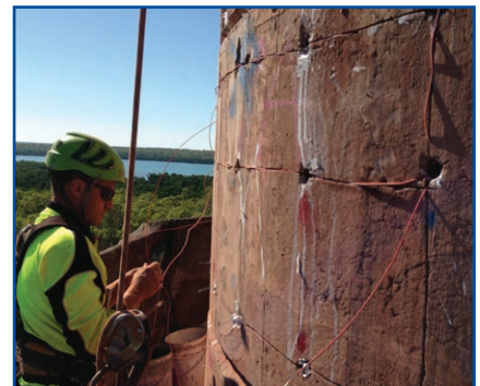
Cape Don Lighthouse, Australia Heritage structure protection
