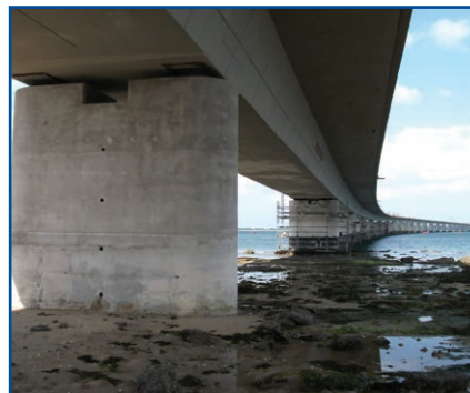
Arosa Bridge, Spain Bridge pier protection
