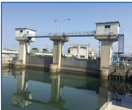
Otanigawa Water Gate, Japan Marine structure protection
