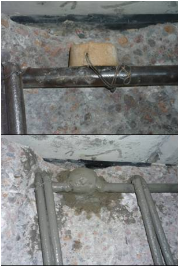
Figure 3. Galvanic anode type B installation procedure, (left) anode tied to the reinforcement as close as practically possible to the edge of the repair and (right) galvanic anode encapsulated in proprietary embedment mortar.
