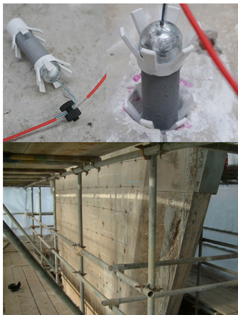
Figure 1. Installation of hybrid anode system to typical reinforced-concrete pier (CPT, 2014)
