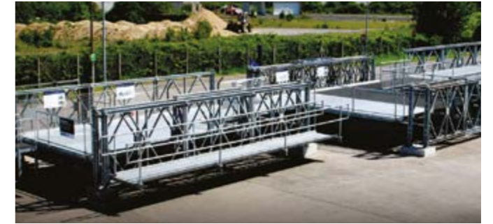
Mabey Bridge's Bridge Park welcomes visitors to see assembled bridges.
