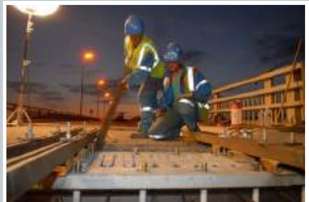
1. WD joint installation tool 2. Detail of anchorage 3. Installing a WP joint
