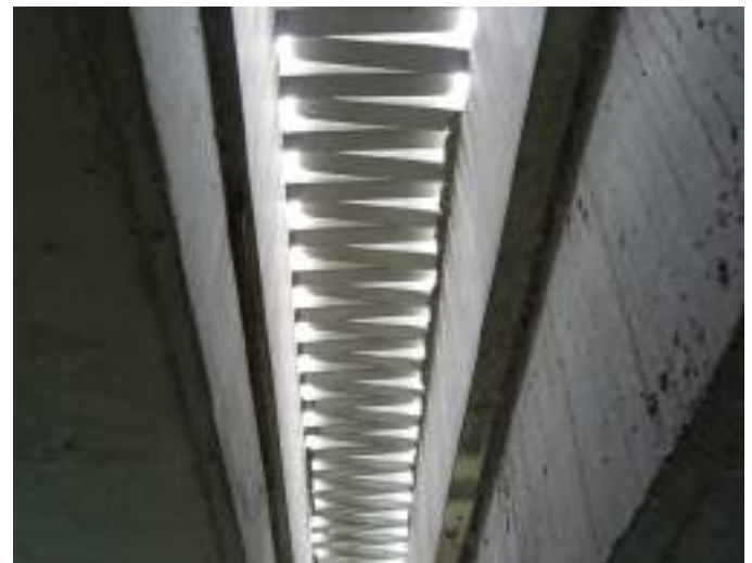
WP joint seen from below
