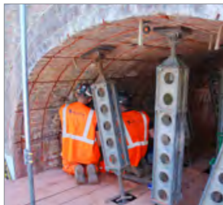
Arch barrel reprofiling
