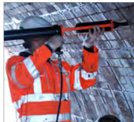
iGap injection process
