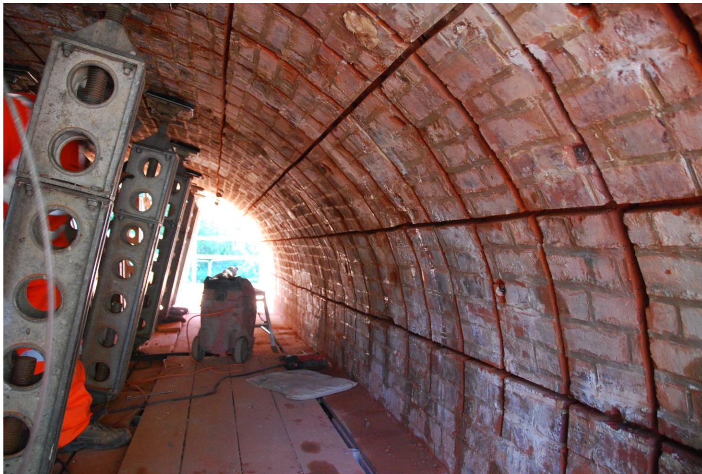
Installation of Betinox stainless steel rebar
