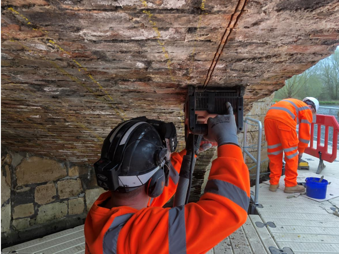
Accurate chasing with no dust and low vibration
