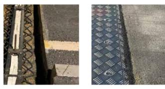
Execution - When it comes to replacement of the joints, damaged areas need to be cut out and all exposed surfaces primed before the Sentinal EMR rails can be lifted into place. Polystyrene shuttering was used before pouring the nosing mortar which was levelled with the road surface. Safetrack, a proprietary anti-skid finish, was then applied.
