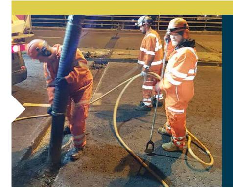
The joint material caters for +/- 20mm movement range (40mm total)
