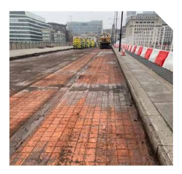
On completion of the concrete repair work the GCP ELIMINATOR<sup>®</sup> waterproofing membrane is applied to provide a minimum dry film thickness of 2mm which equates to 2.8 kg/m<sup>2</sup>
