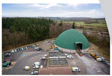
Over 3000 worldwide. 400 in use in the UK and Europe Long service life. Some already 30 years old Factory manufactured timber panels Off-the-shelf design, saves architects costs Diameters: 10m to 50m. Capacities 500 to 25,000 tonnes Natural profile blends into the environment No foundation costs. Concrete walls Salt kept in optimal condition for spreading
