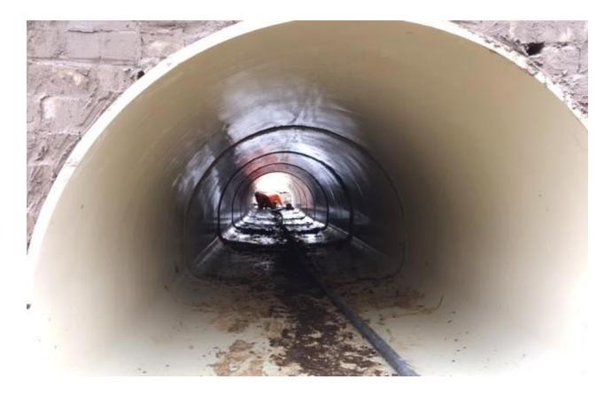
iLine procured the arched GRP segments from our partner Channeline, which were offloaded, installed, grouted, tested and commissioned within a period of 5 days. The resulting status is that the culvert is now structurally sound, has increased flow characteristics, and is designed to withstand all the loadings from the above rail infrastructure, with a design life of 100years.
