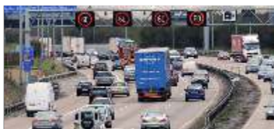
Infrastructure Products – Roads
