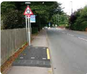
BusPad Ramp Module 750mm wide x 500mm long 65mm high 16.0kg weight
