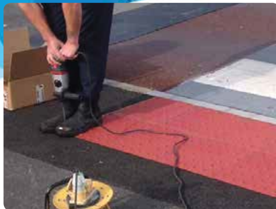
Installation of RediFix tiles
