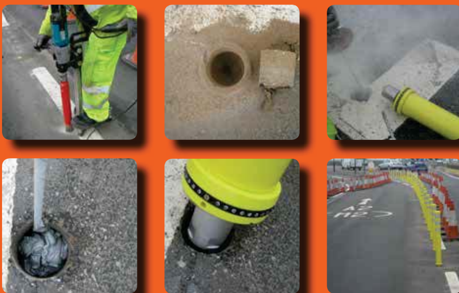
Installing an NS Pole Cone
