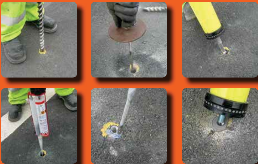
Installing an NSE Pole Cone
