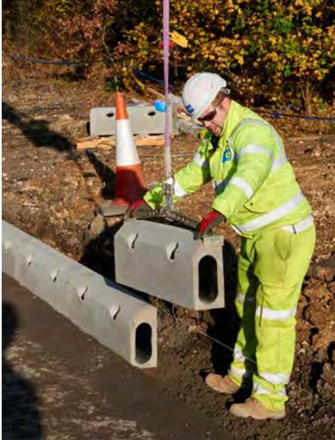
Marshall's supplied 15,000 linear metres of Mono Beany one-piece combined kerb and drainage to the new M1 smart motorway scheme.
