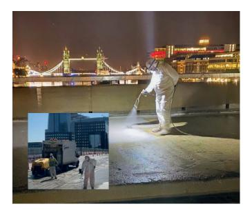
a road bridge, a tack coat (coloured orange) is applied to ensure a strong bond with the asphalt road surfacing.
