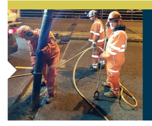
The joint material caters for +/- 20mm movement range (40mm total)
