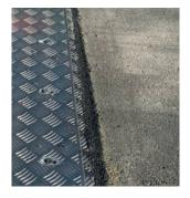
Execution - When it comes to replacement of the joints, damaged areas need to be cut out and all exposed surfaces primed before the Sentinal EMR rails can be lifted into place. Polystyrene shuttering was used before pouring the nosing mortar which was levelled with the road surface. Safetrack, a proprietary anti-skid finish, was then applied.
