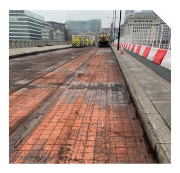
On completion of the concrete repair work the GCP ELIMINATOR® waterproofing membrane is applied to provide a minimum dry film thickness of 2mm which equates to 2.8 kg/m<sup>2</sup>
