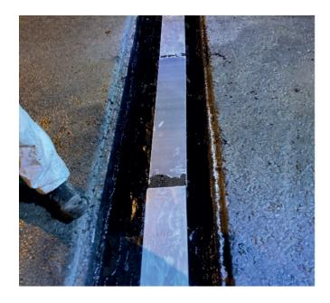
surfaces. After the primer came a first layer of molten PSB, which is a highly flexible material used for tanking the trench. It was applied to the base of the trench, and a galvanised steel plate was placed in the trench. The trench could then be fully tanked out and we installed a drainage channel and rodding box.
