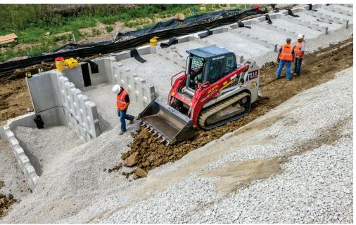
T-WALL® is a gravity retaining wall system, consisting of modular precast concrete units and select backfill. The system is a simple proven solution for grade separation on highway, bridge, railroad, water, commercial applications, and more.
