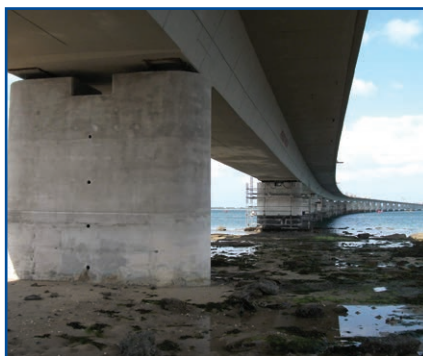
Arosa Bridge, Spain
