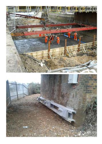
Following the installation of the waling beams; excavation, formwork, steelwork and concrete works could take place safely.
