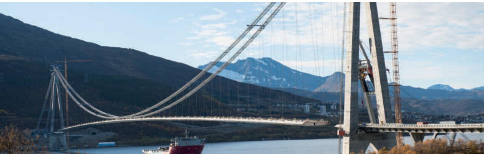
Spiral strand rope and full locked coil rope assemblies have an impressive track record of success in roadbridges. They arrive at the building site ready for installation and therefore allow long span bridges to be constructed within a short period of time.
