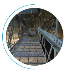
The system replaces traditional suspended scaffolding for under deck working areas on bridges, jetties and ports, providing a safe working platform, designed to suit almost any shape of size of application.
