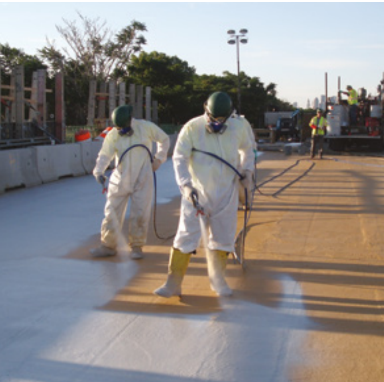
APPLYING SECOND COAT OF ELIMINATOR®
