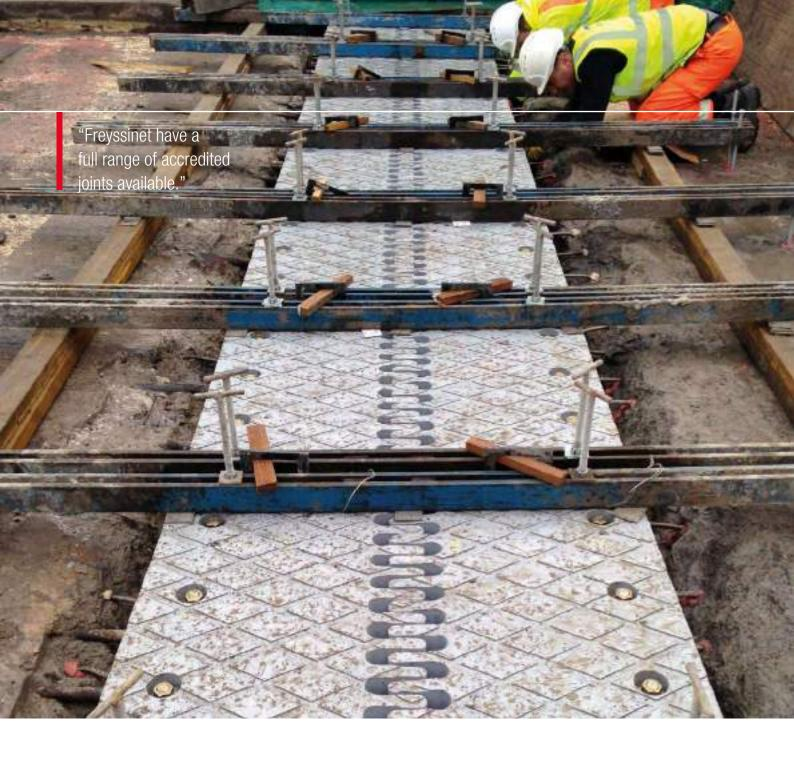
Once the joint anchors are set in place, the concrete is added and allowed to go off. The anchors are then tensioned and the run off surfaces are completed using either a bituminous or cementitious material (Requirements differ depending on where the joint is being installed).
