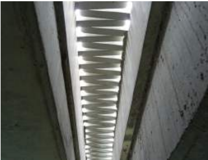
WP joint seen from below
