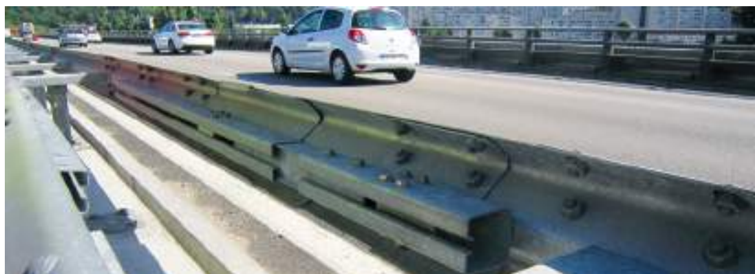
Application on a guardrail
