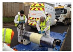
**Patch liners -** Localised no-dig repair using short structural repair sleeves. Very cost-effective. Also available for pressure applications. Up to 1200mm diameter.
