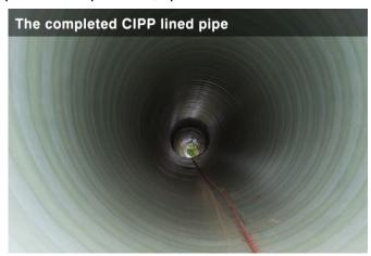
range from 225mm up to 1800mm diameter (up to 30mm thick), over lengths up to 150m. Curing times can be as fast as 1m/minute, depending upon diameter and liner thickness, so the process can be very speedy & much less disruptive than other CIPP methods.
