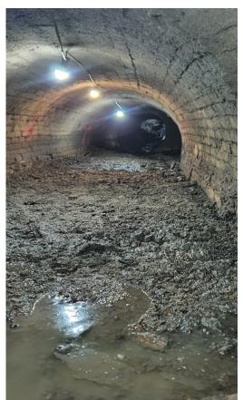
Repairs to brick-arch had previously been carried out. However, the concrete pipes had significant cracks in the crown and was badly deformed caused by settlement of the pipes and there was evidence of scour to the invert. Overall, the structure was considered in danger of possible collapse.
