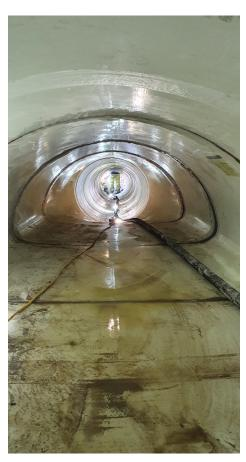
confirmed that due to the manning coefficient of friction an increase of 110% of the original capacity was achieved.
