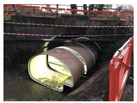
The bridge was constructed of a skew brick-arch section which had previously been repaired, but this was now failing, along with signs of radial cracking occurring. The bridge had been extended in 1971 with a corrugated steel arch which was also now showing signs of corrosion. The structure is shallow,15m long with a flat invert and straight walls, which arches across to a height of 1816mm with a span of 3000mm.
