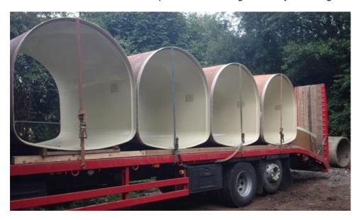
Following the rigorous design process, to ensure that the culvert could withstand the eccentric & unpredictable loadings from the surrounding ground, iLine opted for a traditional, thick section GRP archliner, manufactured by our partner in the Middle-East; manufacture & shipping time was reduced to 5 weeks, enabling a fast-turnaround scheme, much to the delight of the client.
