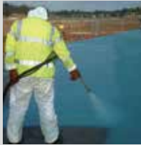
Bridge deck Waterproofing
