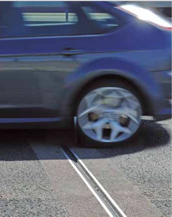
A close up of the BEJ expansion joint system not normally seen by the travelling public.
