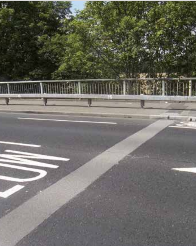
FEBA joint extends across the full length of the carriageway and into the verges.
