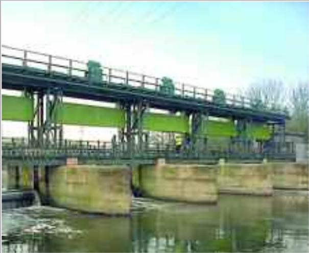
Five river control gates and control system replaced with modern design | Sponden Sluice
