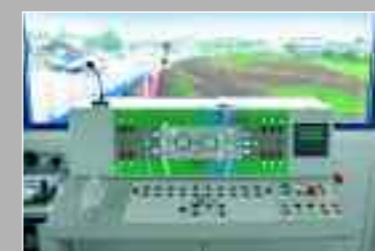
Control panel for Two Mile Bend swing bridge | Gloucester South West Bypass
