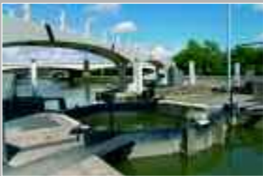
Bow locks two pairs of mitre gates London
