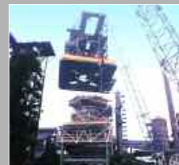
Installation of blast furnace top structure | Scunthorpe
