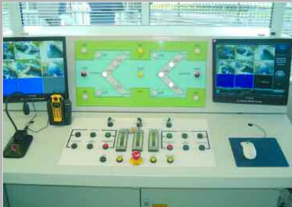
Control panel for Hermitage Lock refurbishment | Cambridgeshire
