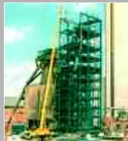
Skip and cage shaft headgear installation Harworth Colliery
