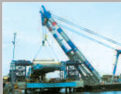
Ro-Ro linkspan installation of top deck Dublin Port
