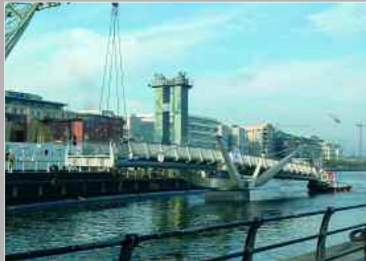
Installation of double leaf pedestrian swing bridge over the River Liffey | Custom House Quay Dublin
