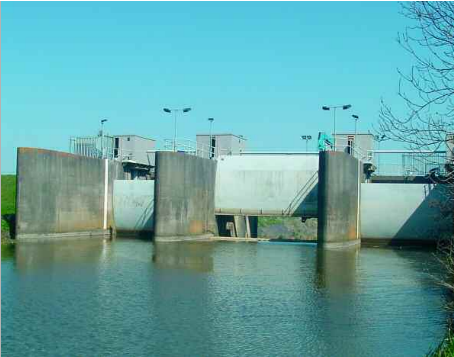
Flood alleviation scheme three radial sluice gates | Leigh Barrier
