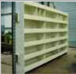
Vertical lift bulkhead gate Ffestiniog hydro-electric power station
