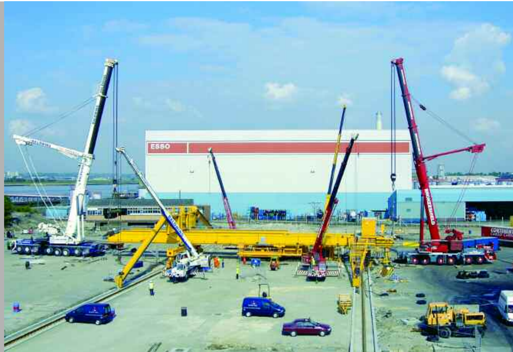
Stage one of erection of crane Purfleet Thames Terminal
