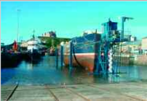
Slipway carriage and winching system | Kilkeel Harbour
