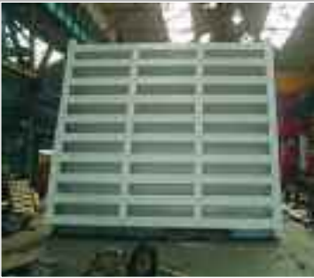
Refurbishment of gate in Qualter Hall works prior to re-installation at site
