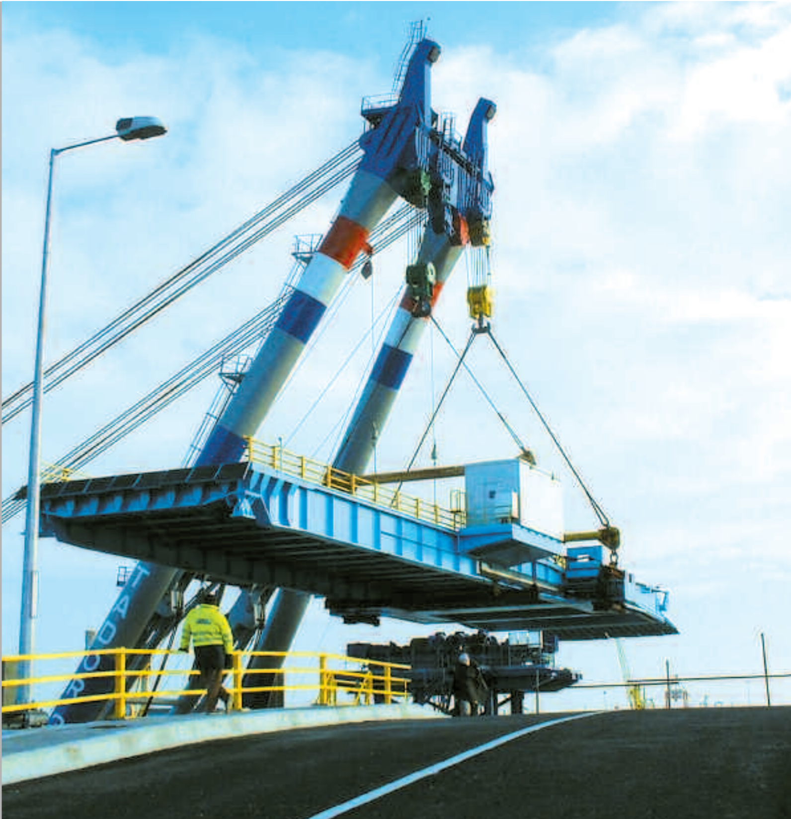
Ro-Ro linkspan installation of top deck | Dublin Port
