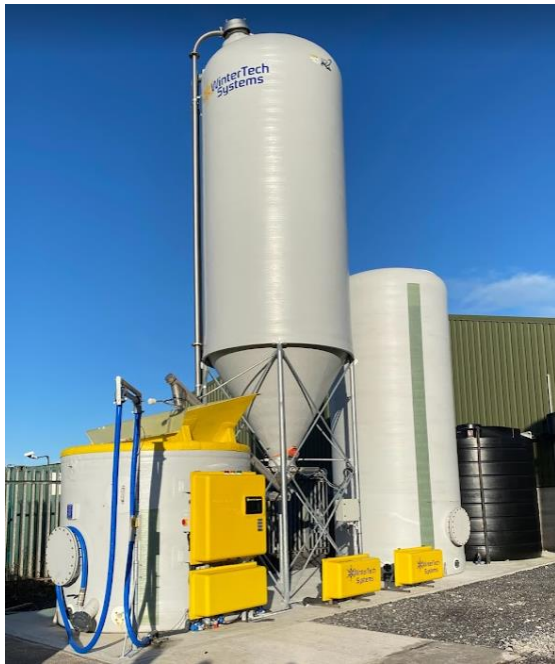
40m 3 silo installation in Mullingar, Ireland
