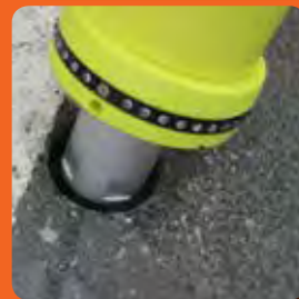
Installing an NS Pole Cone
