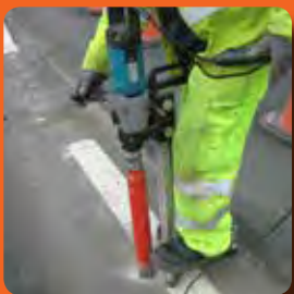
Installing an NSE Pole Cone
