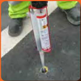
Installing an NSE Pole Cone
