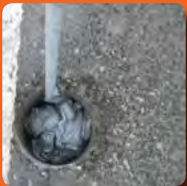
Installing an NS Pole Cone
