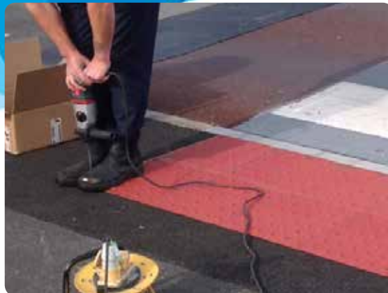
Installation of RediFix tiles
