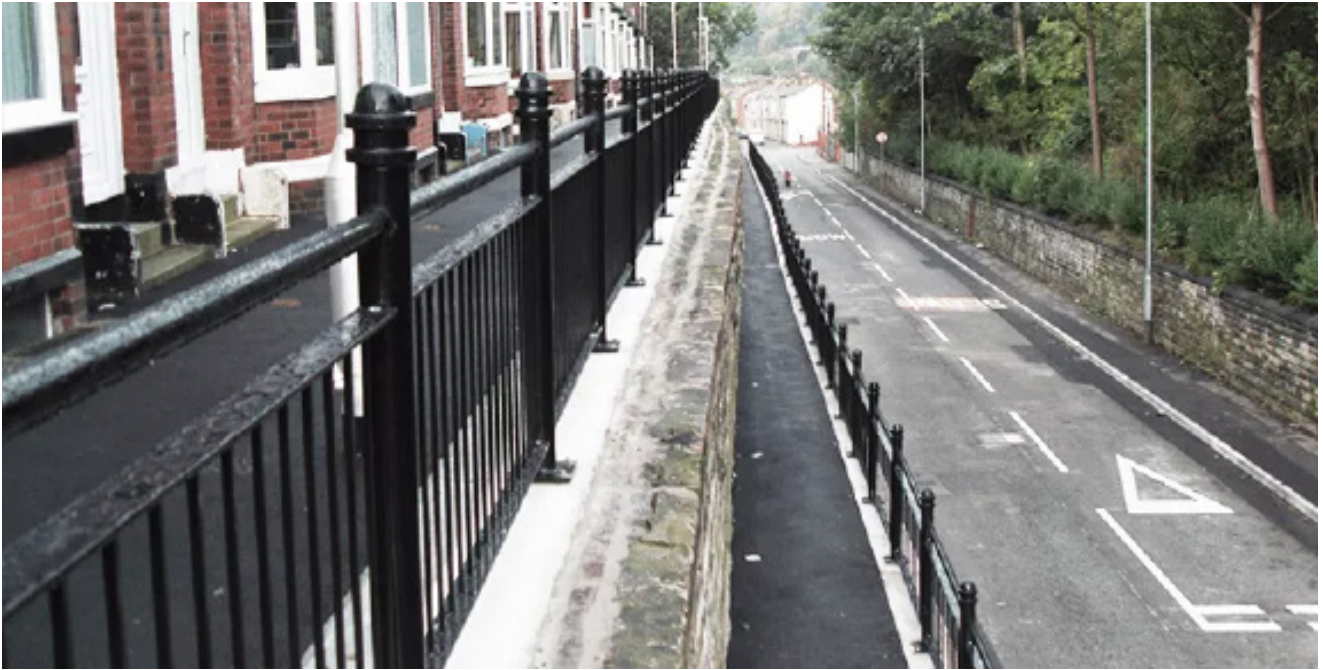
The existing wall was over 100 years old
