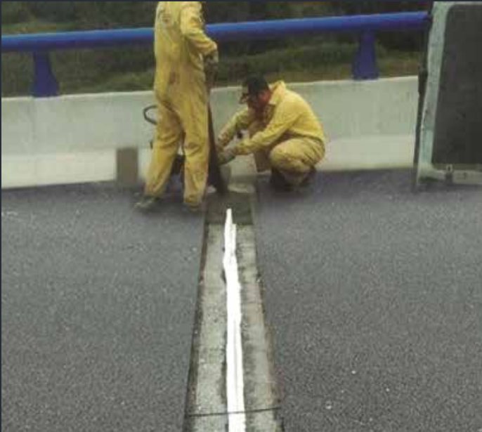
Cutting and removal coating
