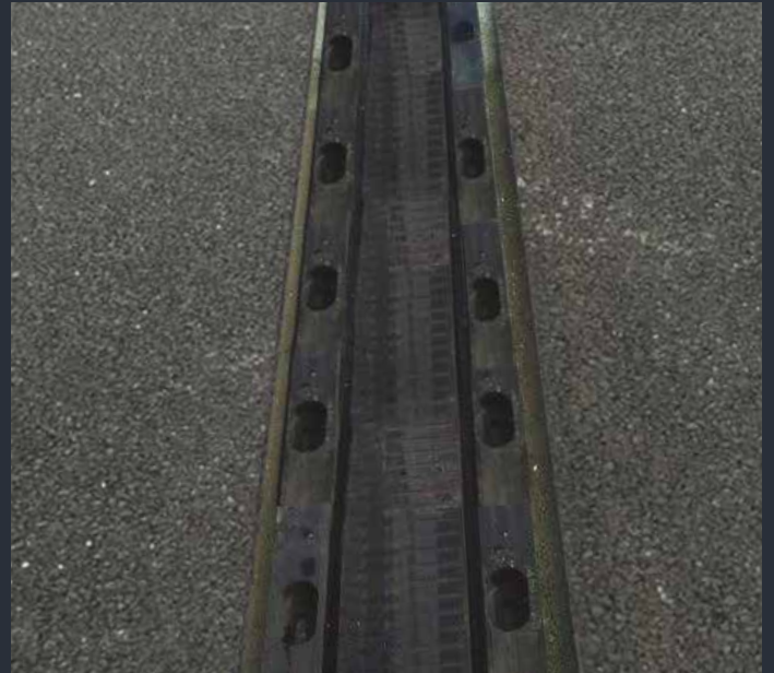
Placement of modules
