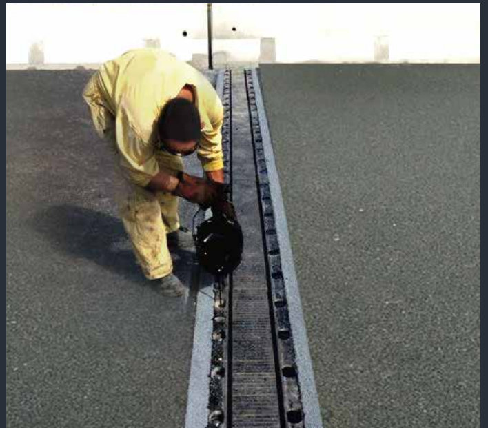
Tensioning the anchors
