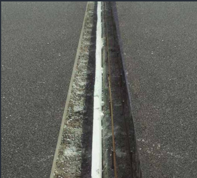
Preparing the anchor fixing
