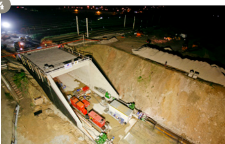
4 - Final sliding and backfilling
