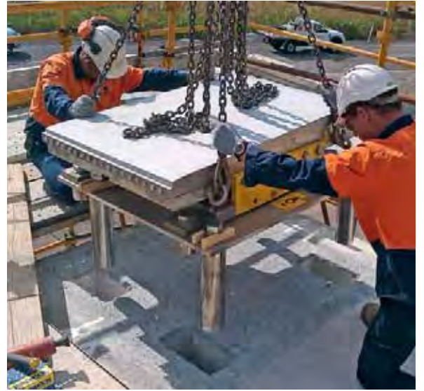
Gerringong Bridge Australia
