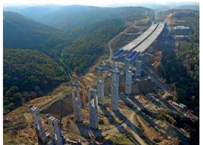
Third Istanbul Bypass Turkey
