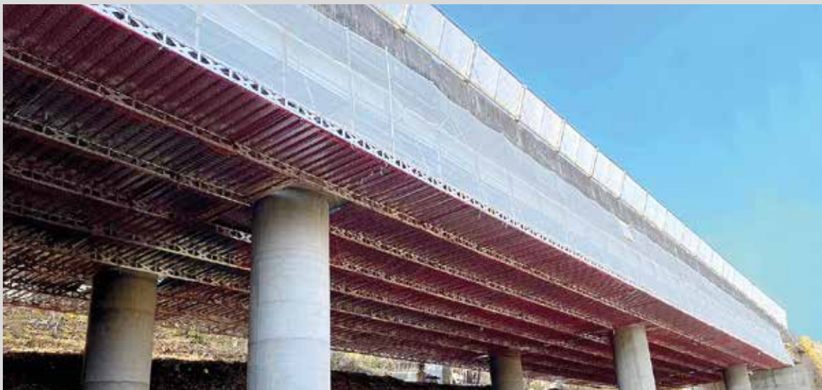
A temporary structure 22 m wide and 250 m long made of 25 cm aluminum beams set up with the FLYRAIL system
