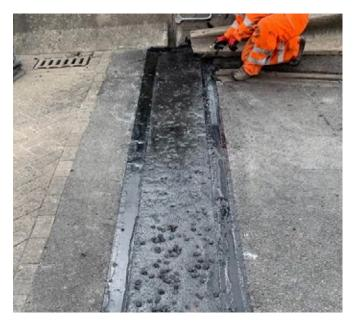
to be free of all dirt and debris. Any concrete repairs are then carried out using specialist repair material.
