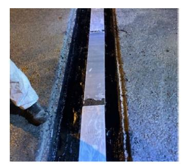
Using the IKO PermaFLASH D300, we plugged the air gap and then applied a primer to all trench surfaces. After the primer came a first layer of molten PSB, which is a highly flexible material used for tanking the trench. It was applied to the base of the trench, and a galvanised steel plate was placed in the trench. The trench could then be fully tanked out and we installed a drainage channel and rodding box.
