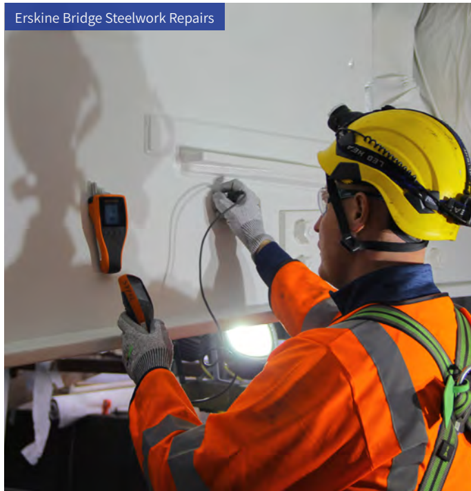
Erskine Bridge Steelwork Repairs
