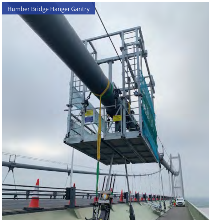
Forth Road Bridge Underdeck Platform
