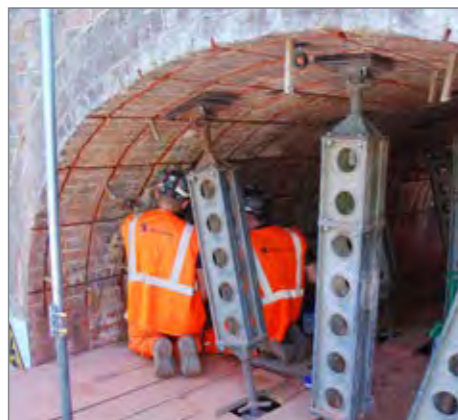
Arch barrel reprofiling
