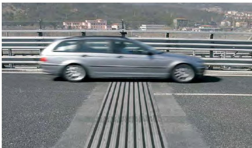
Freyssimod LW joint seam
