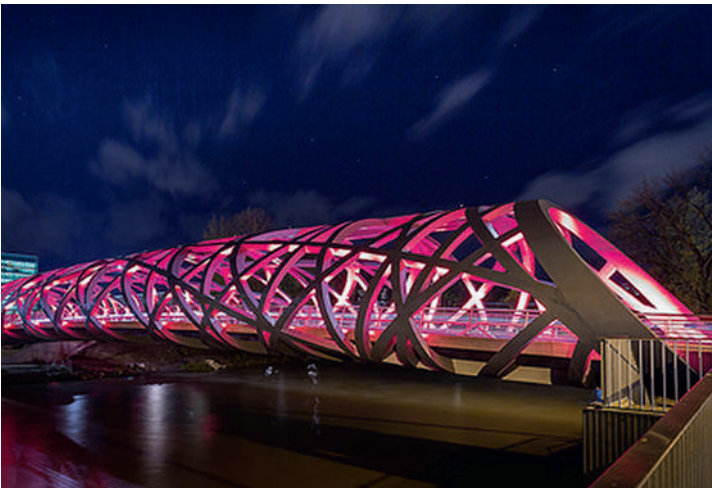
Hans Wilsdorf Bridge Geneva, Switzerland
