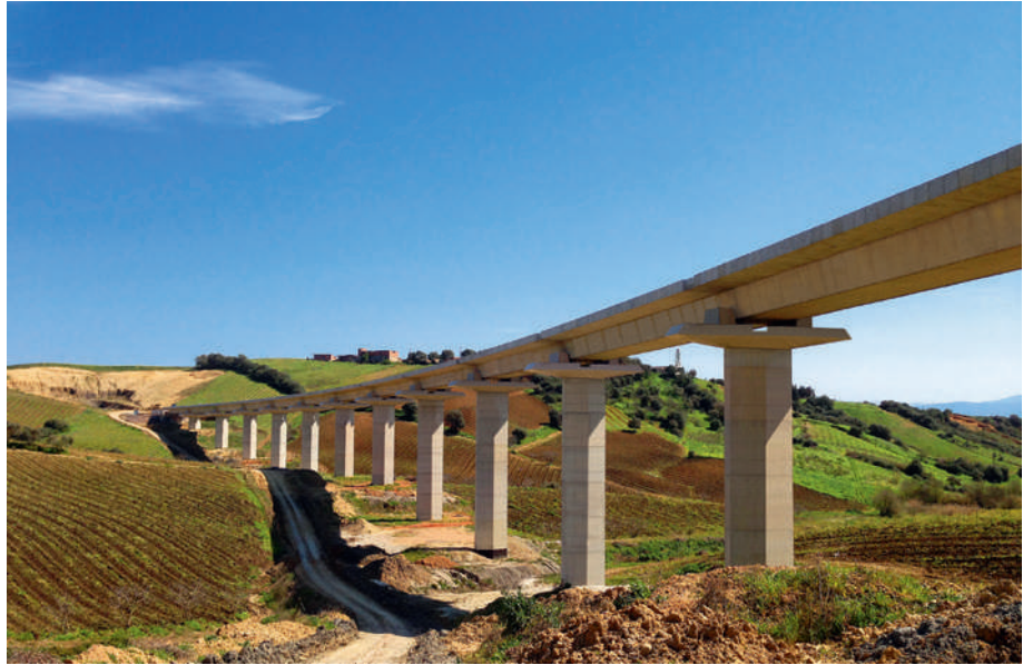
BTZ railway line, Algeria
