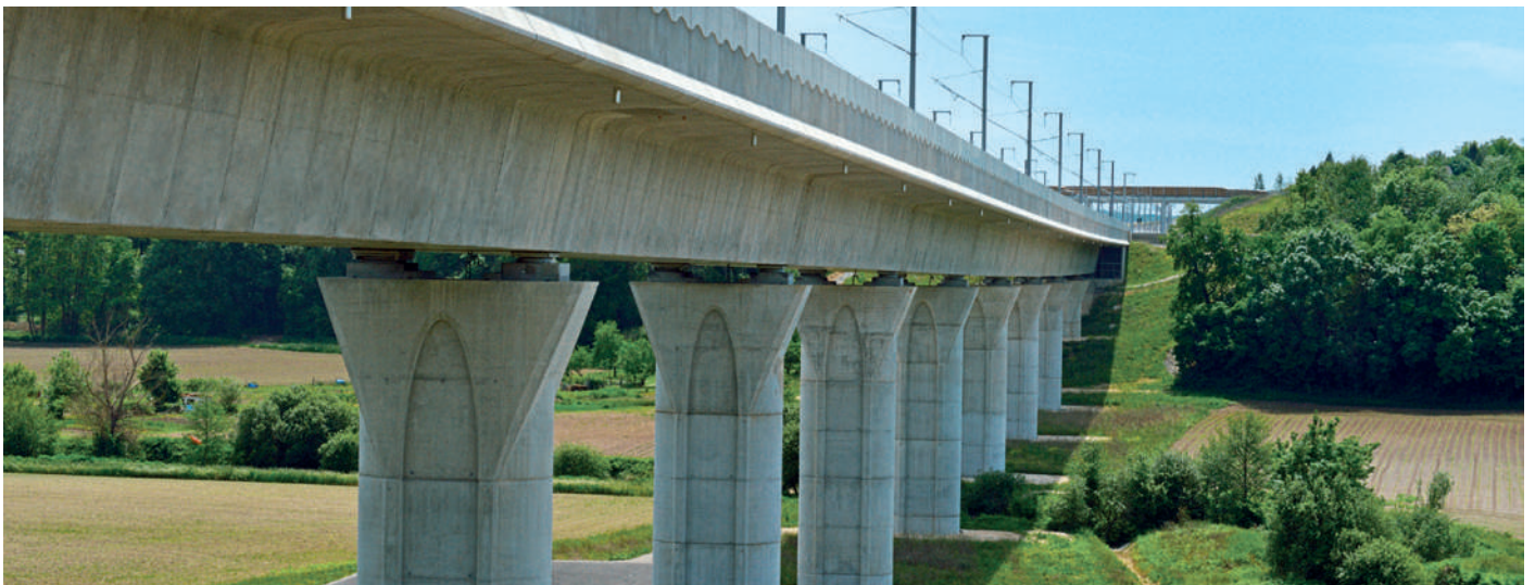
SEA - Tours-Bordeaux high-speed railway line - Boème Viaduct France
