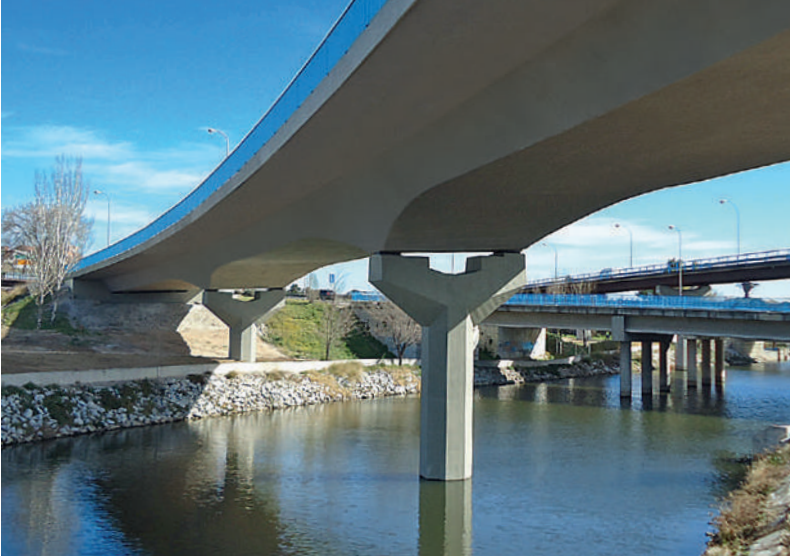
Nudo Sur Bridge on the M-30 Spain
