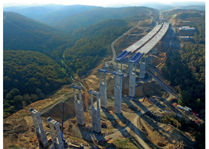
Third Istanbul Bypass Turkey
