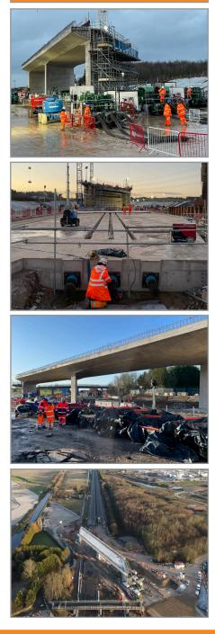
Freyssinet's Autoripage<sup>®</sup> box sliding technique was used on the HS2 Marston Box project and allowed the 85m long, 12,600 tonne Marston Box structure to be slid into place, across the M42, over Christmas 2022. This was a widely recognised success, acclaimed across the HS2 project and in the specialist and general press. Watch the video here.
