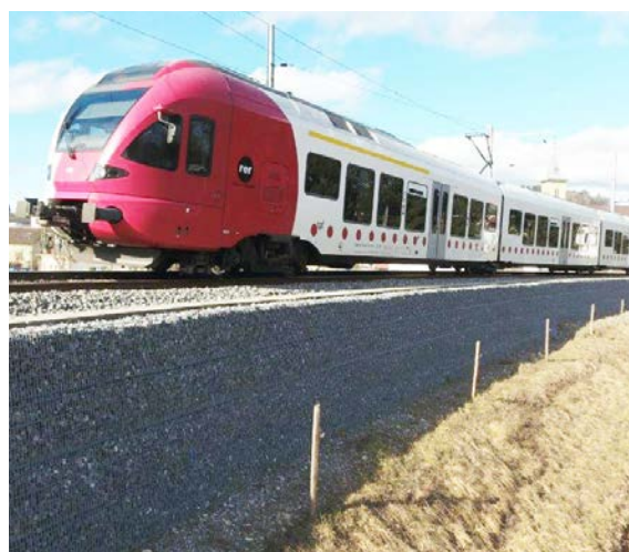
asset BaFix™ 50 stacked in 4 layers using a biaxial grid
