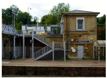
Woolwich Dockyard railway station is in Woolwich in the Royal Borough of Greenwich and has been servicing passengers since 1849. The scheme was to strengthen and refurbish the undercapacity and dilapidated footbridge and associated staircases to provide a maintenance free design life of a minimum 15 years.
